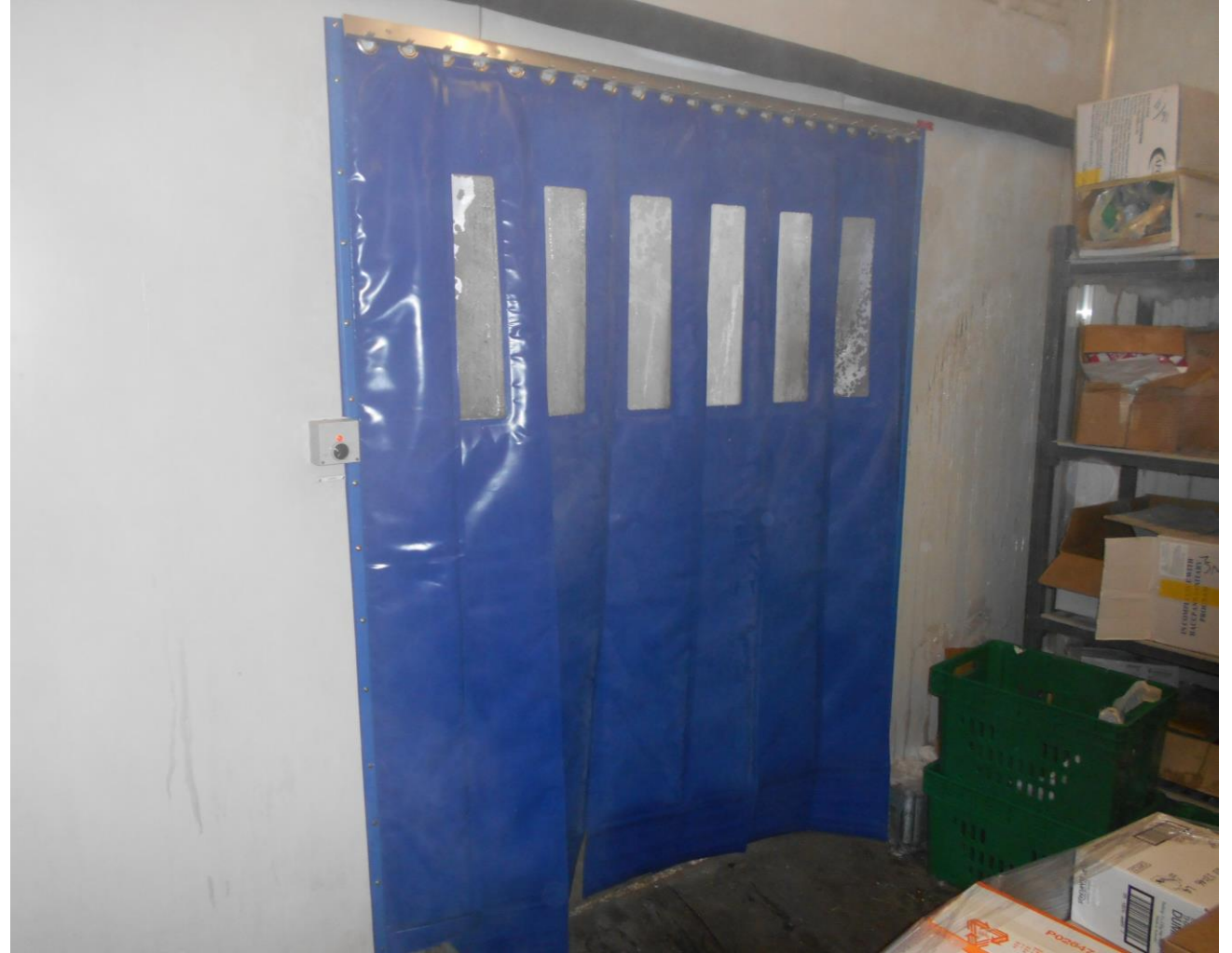
Post Installation Cool Room Door – Internal View
