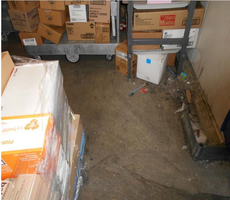
Post Installation LT Room – No ice build up on entry door
