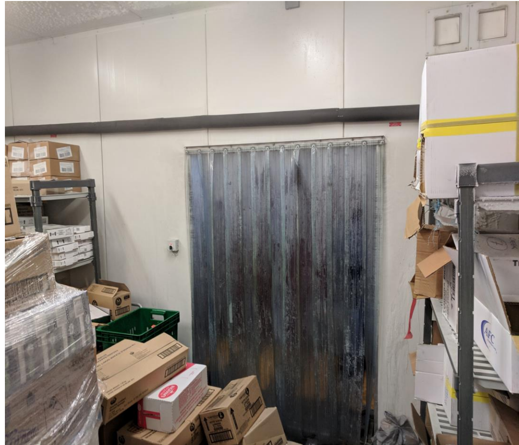
Pre Installation Cool Room Door – Internal View
