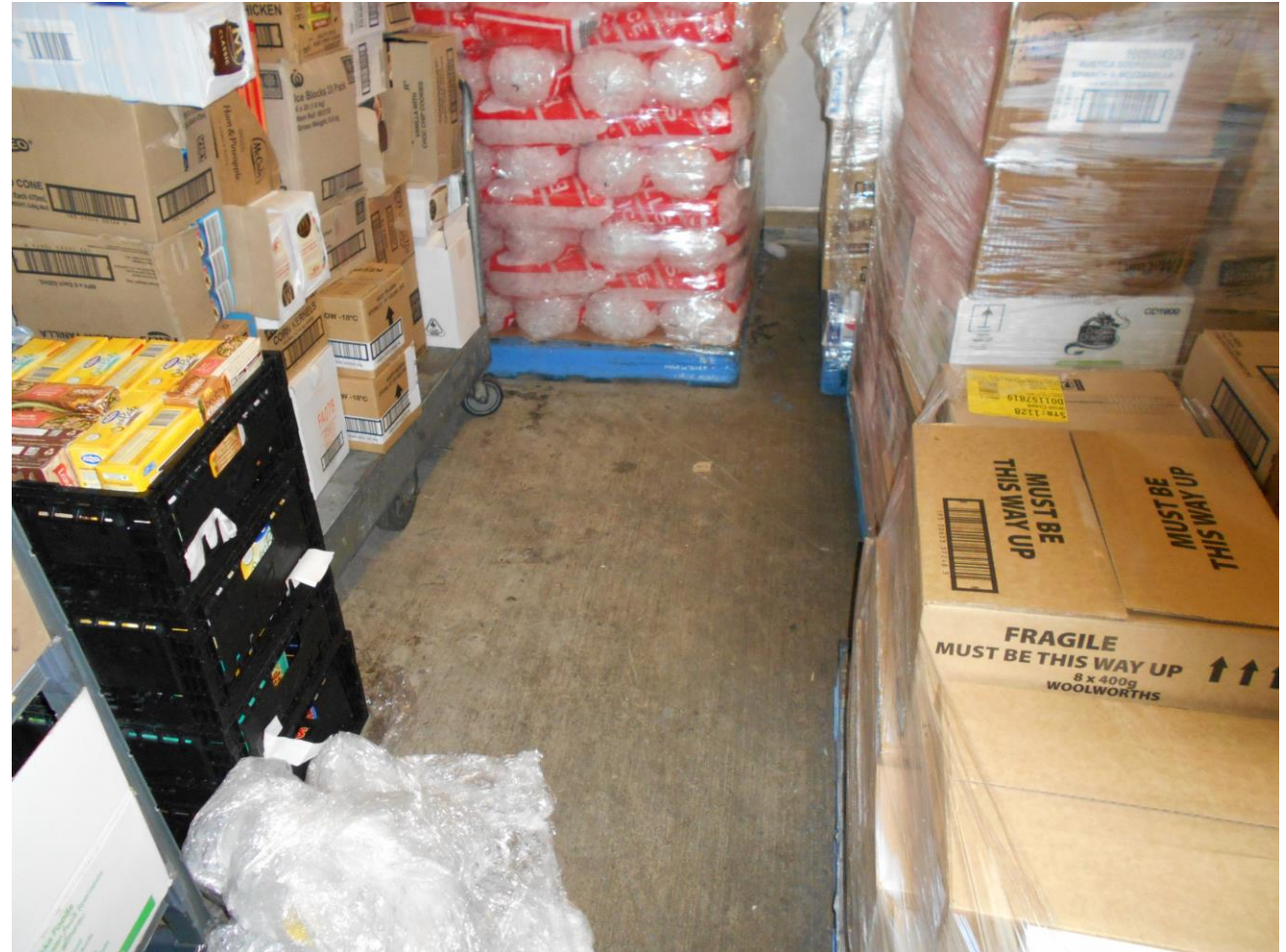
Post Installation LT Room – No Ice build up on Floor – significantly reducing slip hazards
